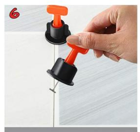
6: Take out the leveler along the edge of the gap, it can be recycled
