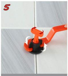
5: Rotate the adjustment cover counterclockwise, and then rotate the T-type leveler by 90° to make it parallel to the tile gap
