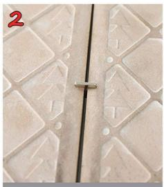
2:90°rotating T-type leveler Fix it at the point of 2 tiles
