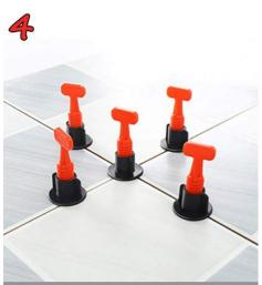
4:Wait 4-6 hours, take out the leveler when the tile glue and not completely solidified
