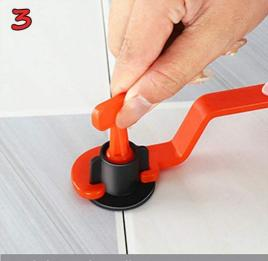
3:Tighten the adjustment cover clockwise by hand or a wrench to make the weo tiles on the same level
